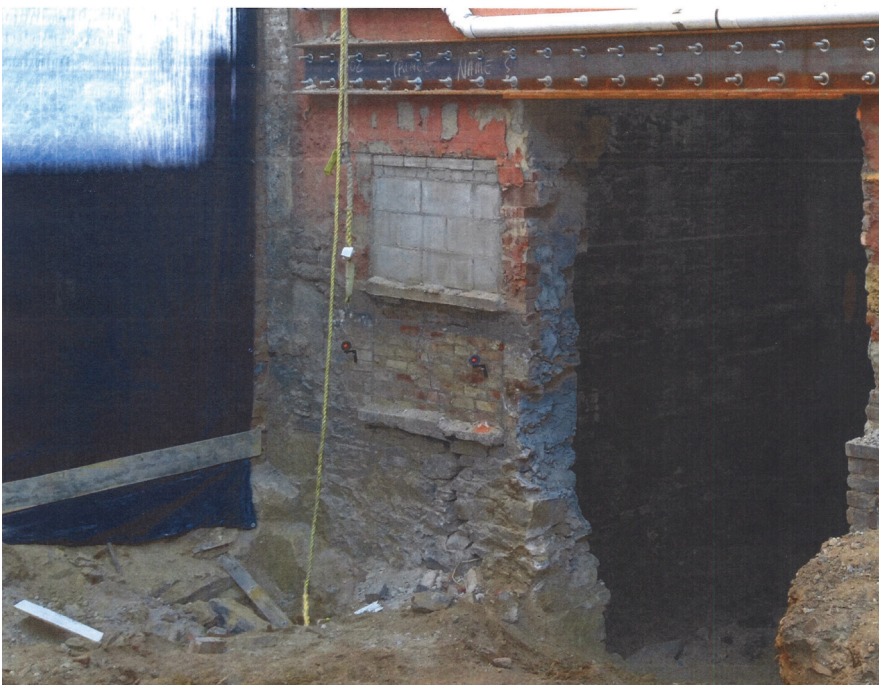
Figure 2. Prisms monitoring large crack in a building.
